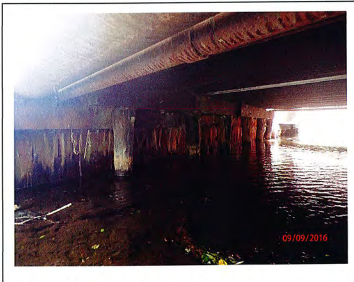
W. Abutment, N. Culvert
