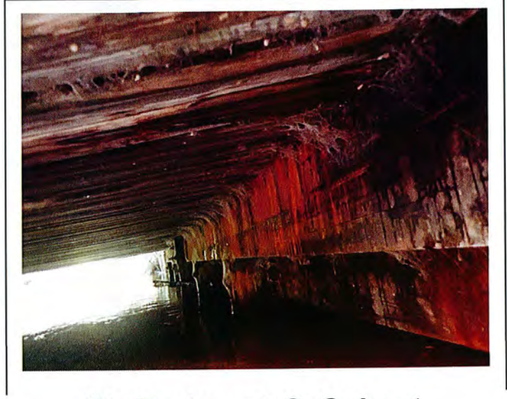
W. Abutment, S. Culvert
