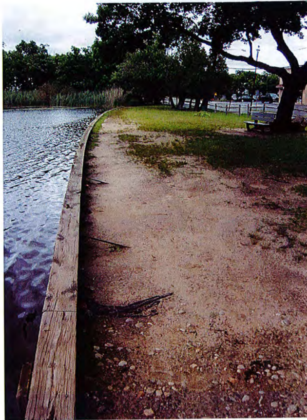
Photo # 3: Exposed steel tie-backs
