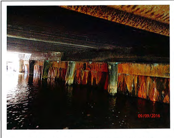
W. Abutment, N. Culvert
