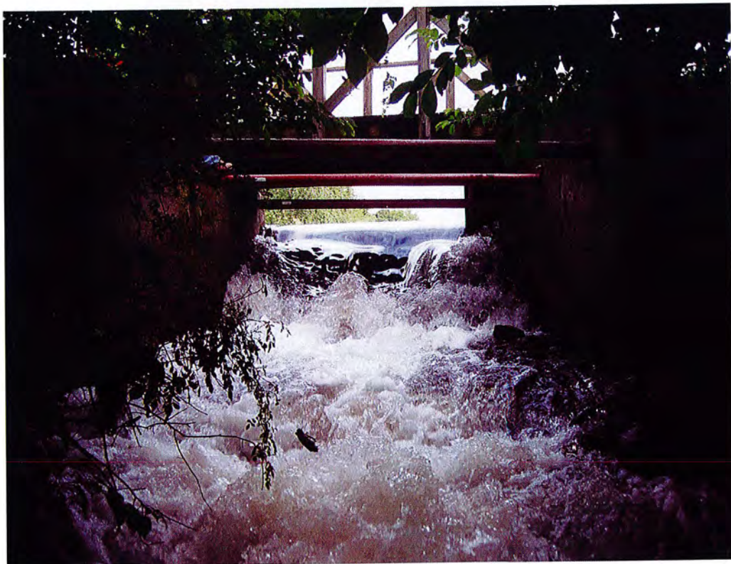
Photo # 4: Willow Lake spillway
