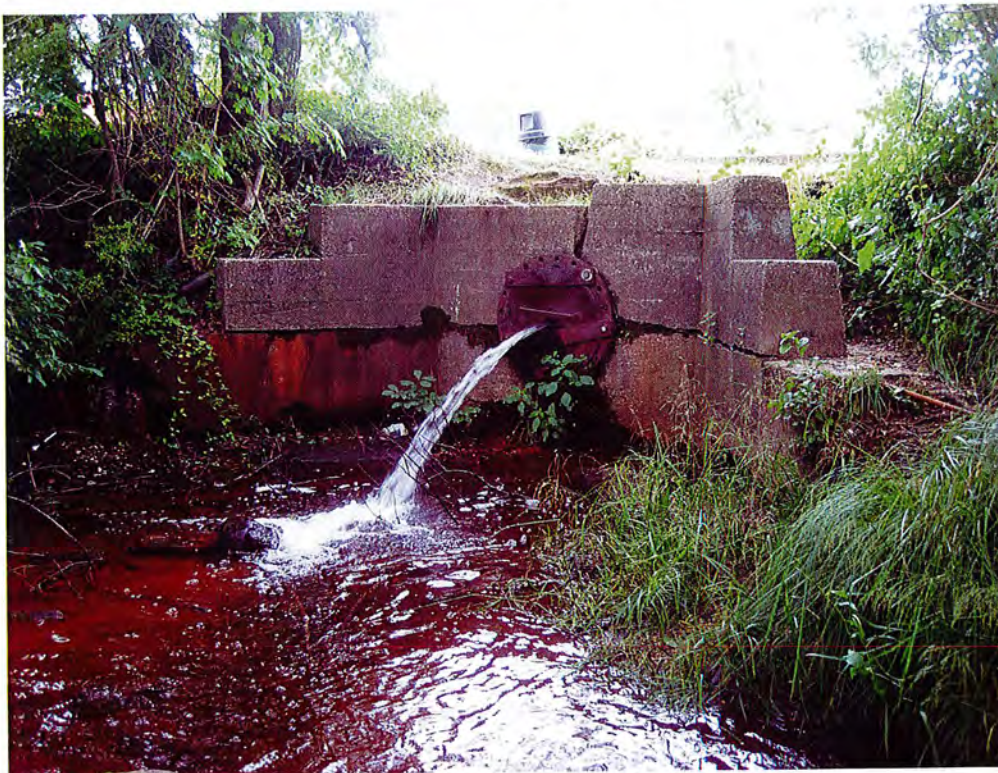
Photo # 6: Low level outlet
